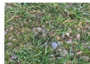
parking terre-pierre enherbé
